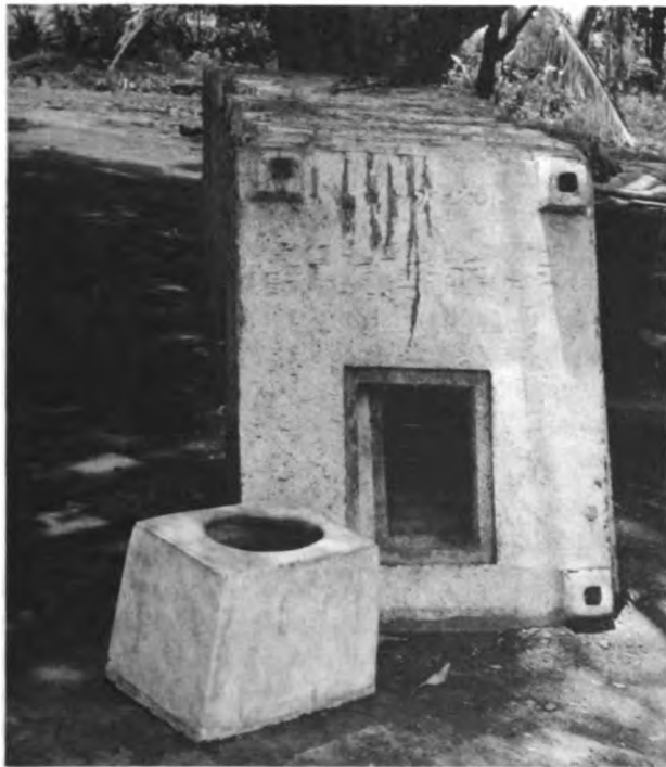
Newly made sanitary latrine base slabs are ready for distribution to villagers in Nicaragua. These slabs are placed over a pit and a seat box is fitted over the opening. Wooden covers are placed over the seat opening when the latrine is not in use.
