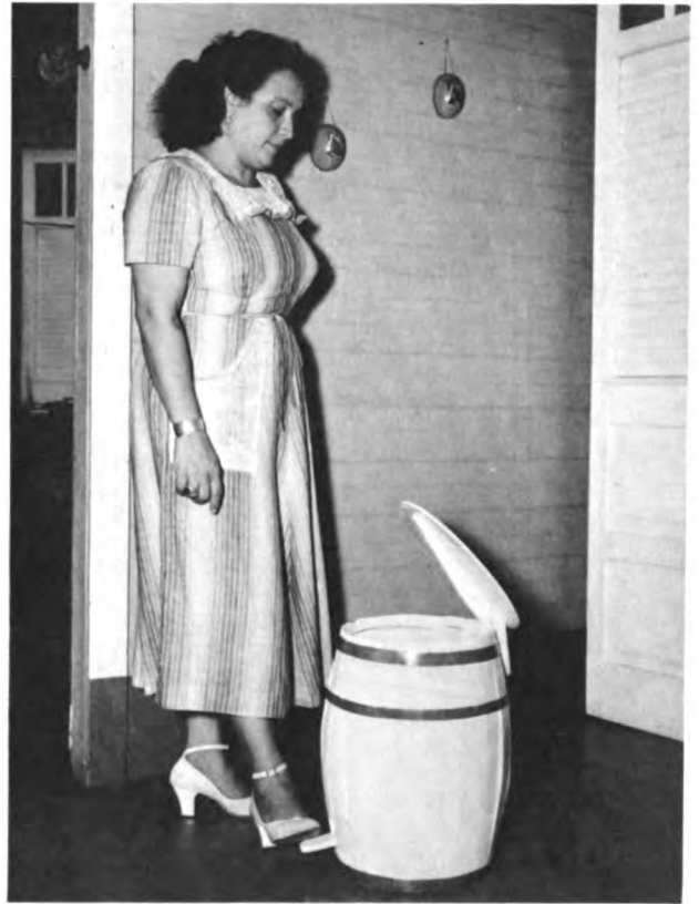
Garbage containers can be made of many easily available materials. This homemaker in Puerto Rico has made one of an old nail keg. She has put a tight-fitting lid on it to keep out flies.
