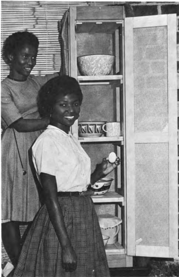
These two iceless coolers help keep perishable foods from spoiling so rapidly. They both work on the principle of evaporation. The one on the left was built by two
