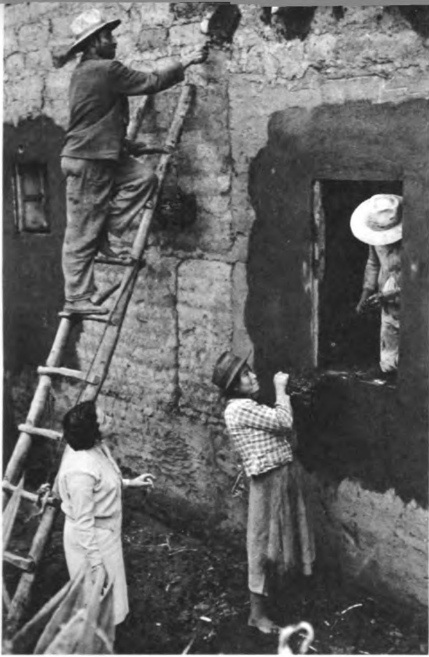
On the home improvement worker's advice, this family in Ecuador repaired the cracks in the walls of their home before they put on a new coat of plaster.
