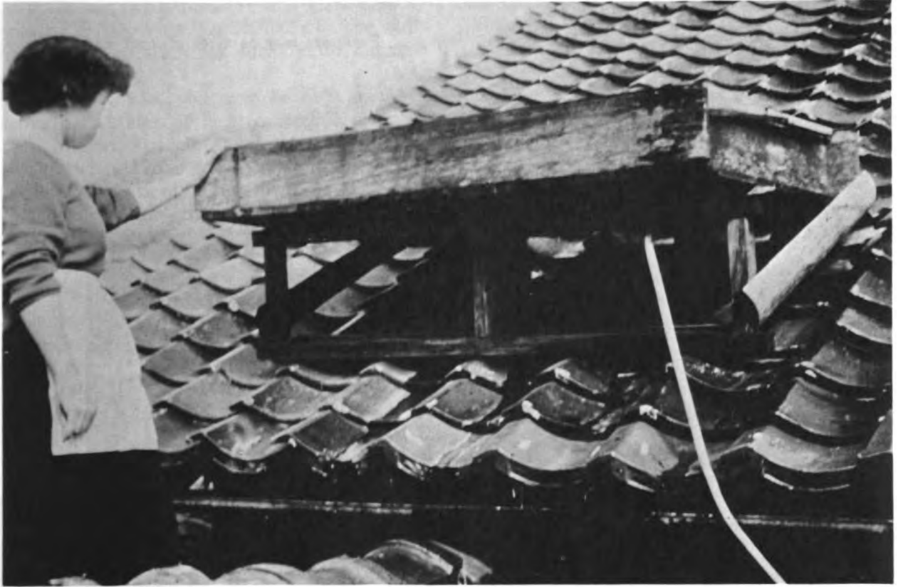
Solar water heaters in Japan catch rainwater from the roof and hold it for the sun to heat. It is then piped into the home.
